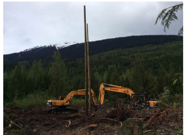
Photo 7. Pole installation work in Segment 1 (May 23, 2014).
