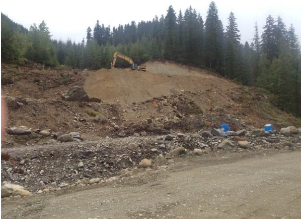
Photo 1. Bulk excavation of the BDRHEF downstream portal location (May 23, 2014).
