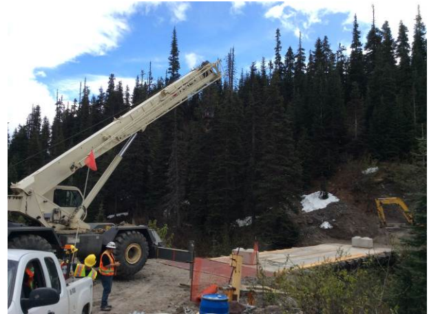
Photo 5. Keyhole Bridge re-enforcement works. (May 24, 2014).
