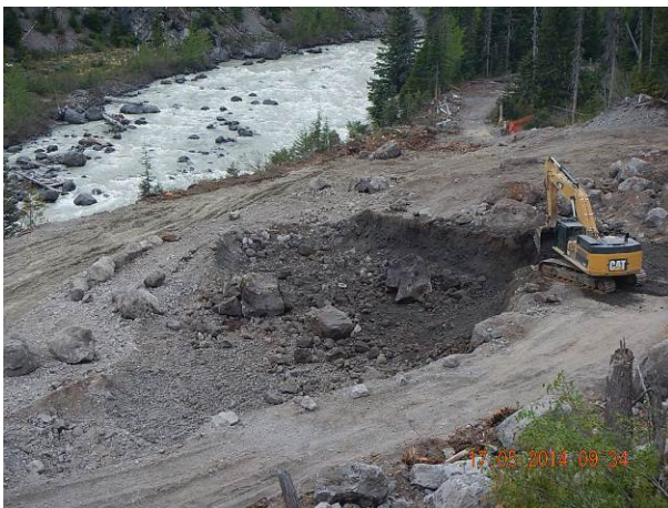
Photo 3. Bench excavation at the ULRHEF powerhouse area. (May 17, 2014).
