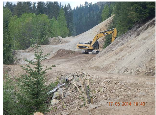
Photo 4. Road construction along the Truckwash Creek Bypass road. (May 17, 2014).
