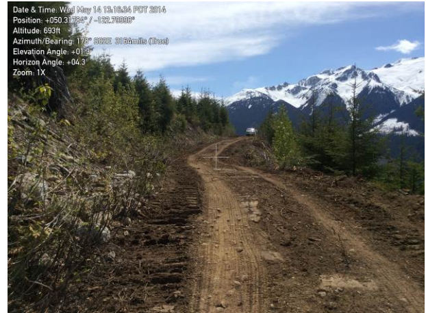
Photo 6. Pebble Branch D.1 access road following access road upgrades (May 14, 2014).
