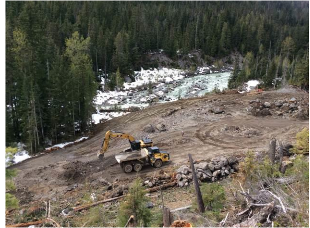
Photo 4. Stripping and grubbing activity at the ULRHEF powerhouse location. (May 9, 2014).
