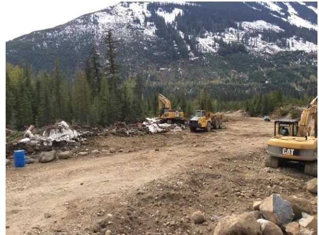
Photo 2. Stripping and grubbing activity at the BDRHEF powerhouse location. (May 3, 2014).
