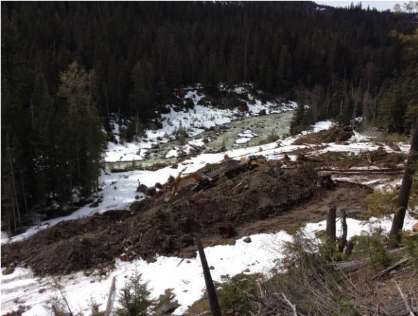
Photo 3. Stripping and grubbing material from the ULRHEF powerhouse work area. (May 3, 2014).
