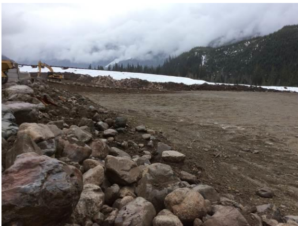
Photo 3. Overview of the grading works at the 38km laydown area. (April 16, 2013).
