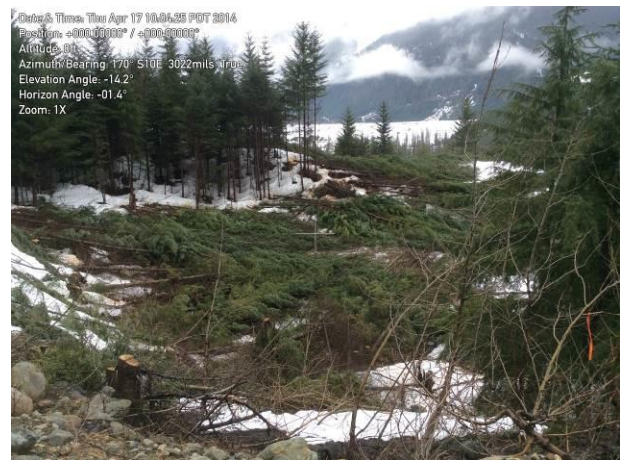
Photo 4. Hand falling at the future Construction Camp (middle) location. (April 17, 2013).
