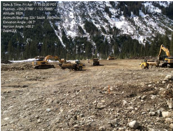
Photo 1. Overview of the grading works at the 38km laydown area. (April 11, 2013).
