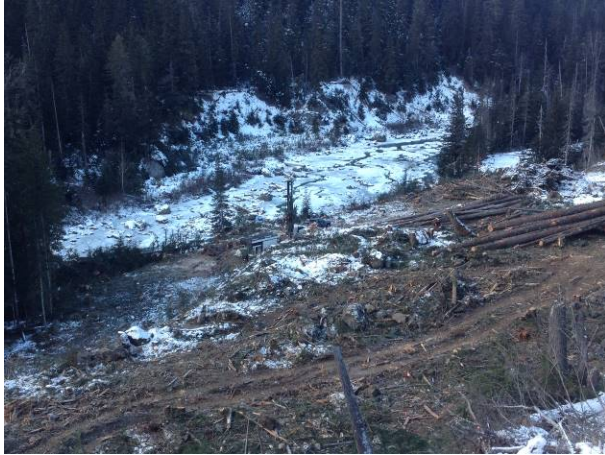
Photo 1. Drilling equipment in operation and site conditions at the ULRHEF powerhouse (Dec 8, 2013).
