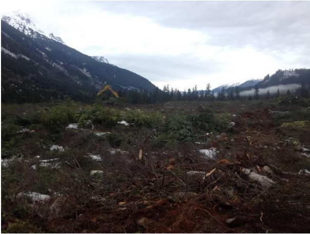
Photo 3. Piling trees with an excavator at the construction camp. (Nov 27, 2013).
