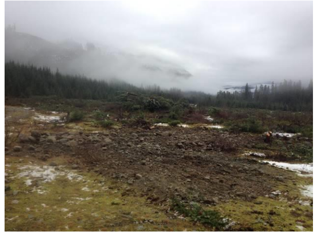
Photo 4. New test pit at the construction camp. (Nov 28, 2013).
