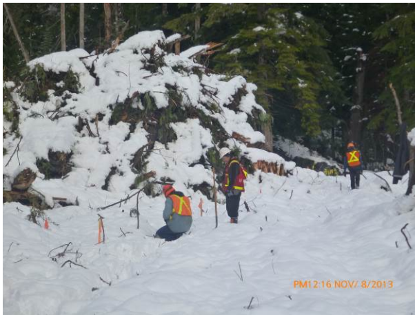
Photo 3. Seismic survey work being conducted in the presence of the archeology monitor at the ULRHEF intake area (Nov 8, 2013).
