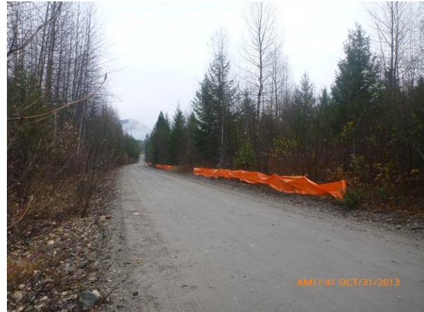
**Photo 4. Gaps installed in the visual barrier fencing installed to protect the adjacent wetland areas along the Lillooet River FSR (Oct. 31, 2013).**
