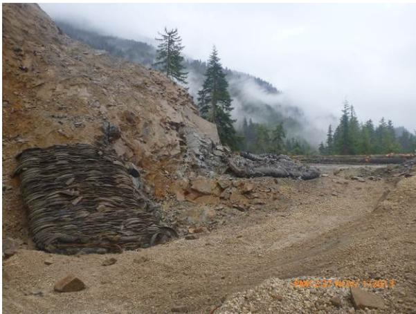
**Photo 1. Blast mats used during blasts within 500m of Grizzly Bear Class 1 habitat (suitable summer and fall forage; ULL-GB05) and with 500m of Mountain Goat UWR (UL11) at the west heading of the Truckwash Creek FSR realignment (Nov 1, 2013).**
