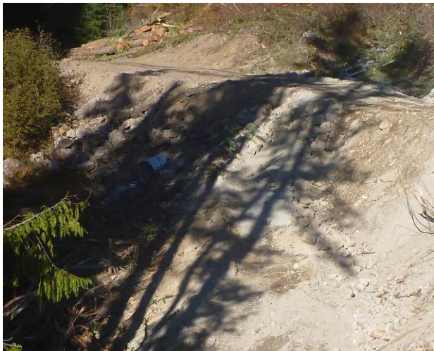
Photo 1. Road base backfill placed over 1600mm culvert at Stn. 1+430 (Oct. 25, 2013).
