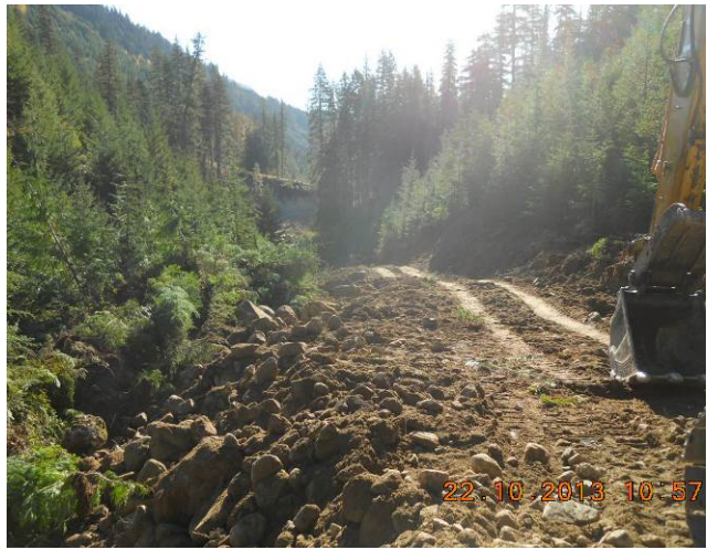
Photo 2. Clearing and grubbing within 500m of Grizzly Bear Class 1 habitat (suitable summer and fall forage; ULL-GB05) at the east heading of the Truckwash Creek FSR realignment (Oct. 23, 2013).
