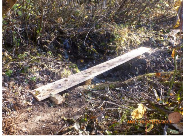
Photo 4. Boardwalk constructed over sections of flowing water (Oct. 25, 2013).
