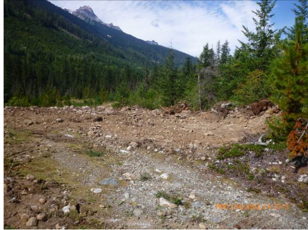
Photo 2. Production Well site #2 clearing. (Aug. 23, 2013)
