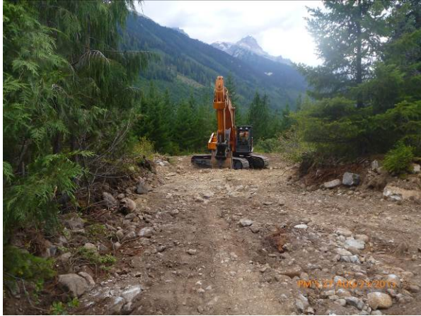
Photo 1. Production Well site #1 clearing. (Aug. 23, 2013)
