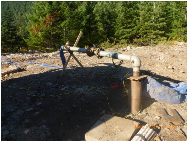
Photo 5. Production well testing setup. (Sept. 11, 2013)
