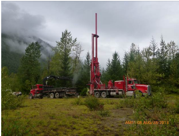
Photo 3. Monitoring well drilling. (Aug 28, 2013)
