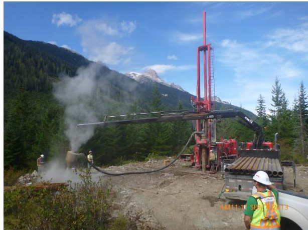
Photo 4. Production well drilling at site #1. (Sept. 4, 2013)
