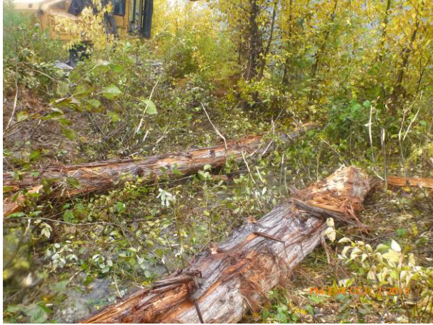
Photo 5. One example of a temporary crossing installed by the feller buncher to cross an open channel without impacting the stream banks or substrate (Oct. 7, 2013).
