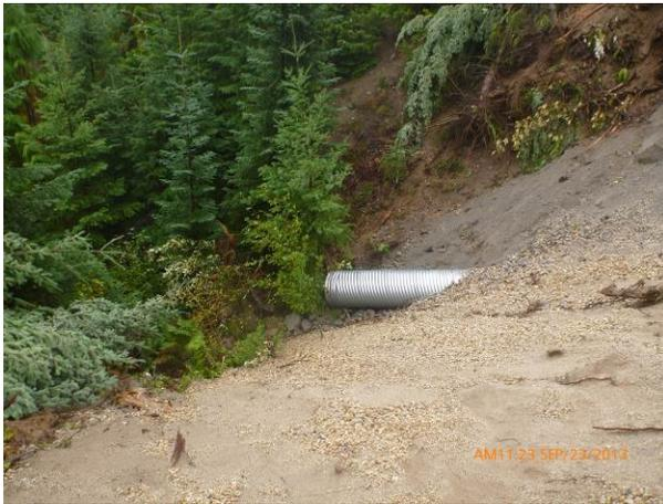
**Photo 1. Culvert installed within dry ephemeral channel (Stn. 2056.0 – Sept. 23st, 2013)**
