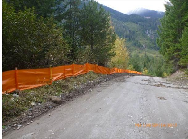
**Photo 4. Visual screen installed along Lillooet River FSR >30m from an identified wetland (Sept. 24, 2013).**
