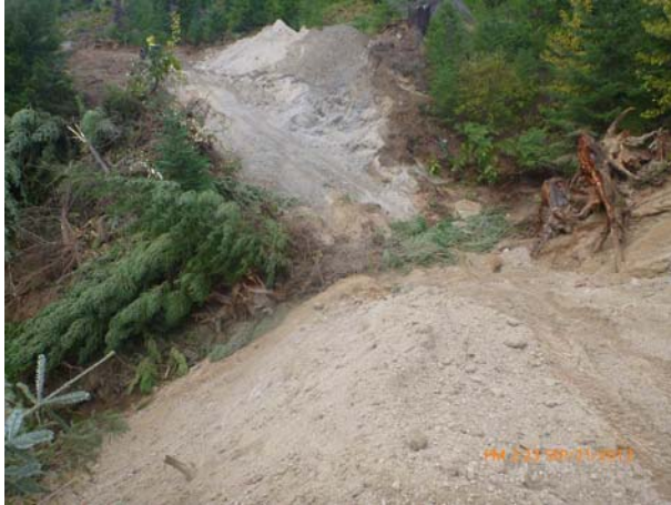
Photo 1 Temporary ford of dry ephemeral channel (Stn. 2056.0 – Sept. 21st, 2013)
