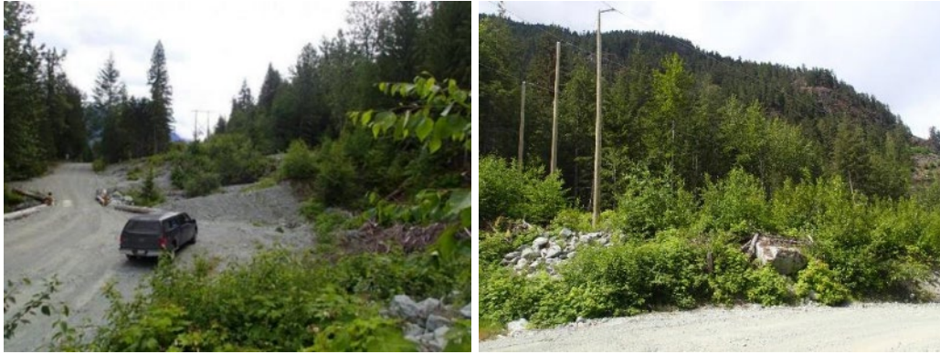
Figure 28. Vegetated screen along the transmission line at ULH-MAMCM17, assessed on June 6, 2018.
