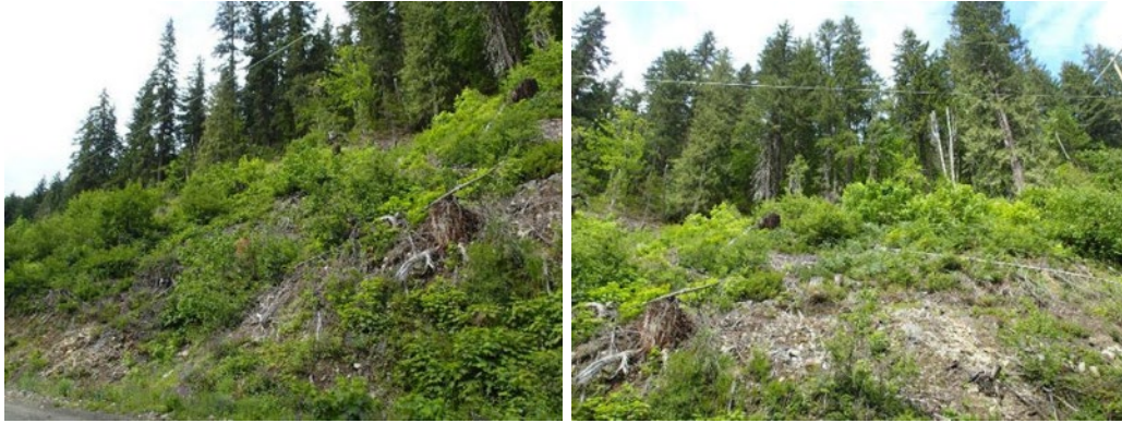
Figure 19. Vegetated screen along the transmission line at ULH-MAMCM10, assessed on June 14, 2018.
