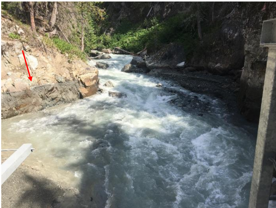
Figure 20. Boulder intake displaying the successful removal of bedload from the headpond post sediment management on August 9, 2019. Red arrow is a visual representation of the height of sediment pre-sediment management activities.
