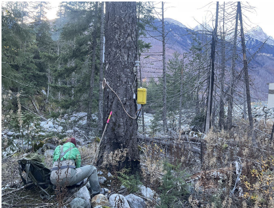
Figure 32. Looking at BDR-DVAT on October 27, 2023.
