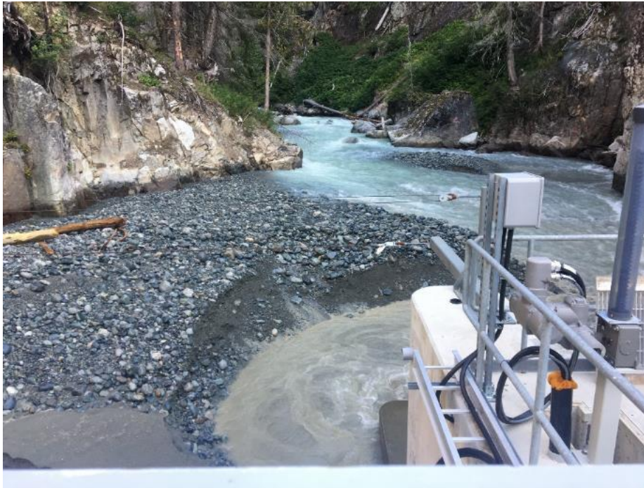
Figure 19. Boulder intake displaying naturally-accumulated bedload in the headpond prior to routine sediment management on August 9, 2019.
