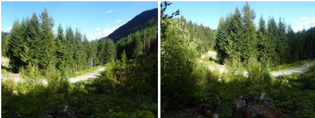
Figure 53. Vegetated screen along the transmission line at ULH-MAMCM28, assessed on August 25, 2020.
