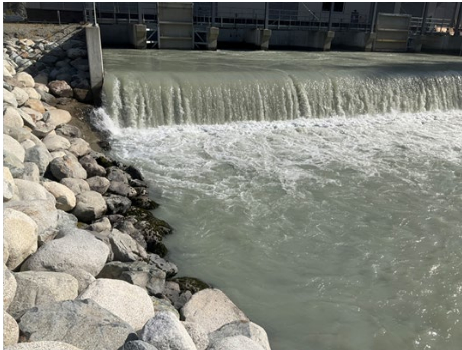
Figure 10. Looking upstream at ULL-TAILWQ on October 06, 2023.
