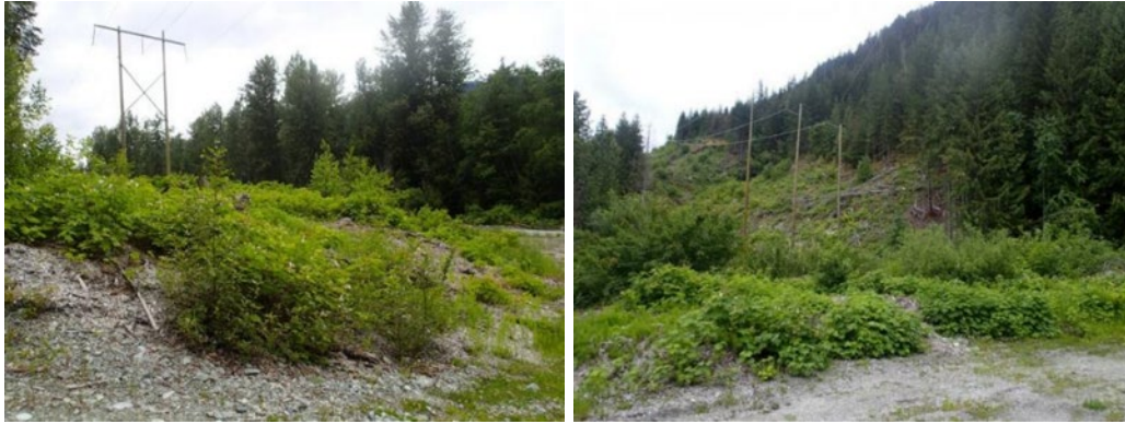
Figure 31. Vegetated screen along the transmission line at ULH-MAMCM19, assessed on June 6, 2018.
