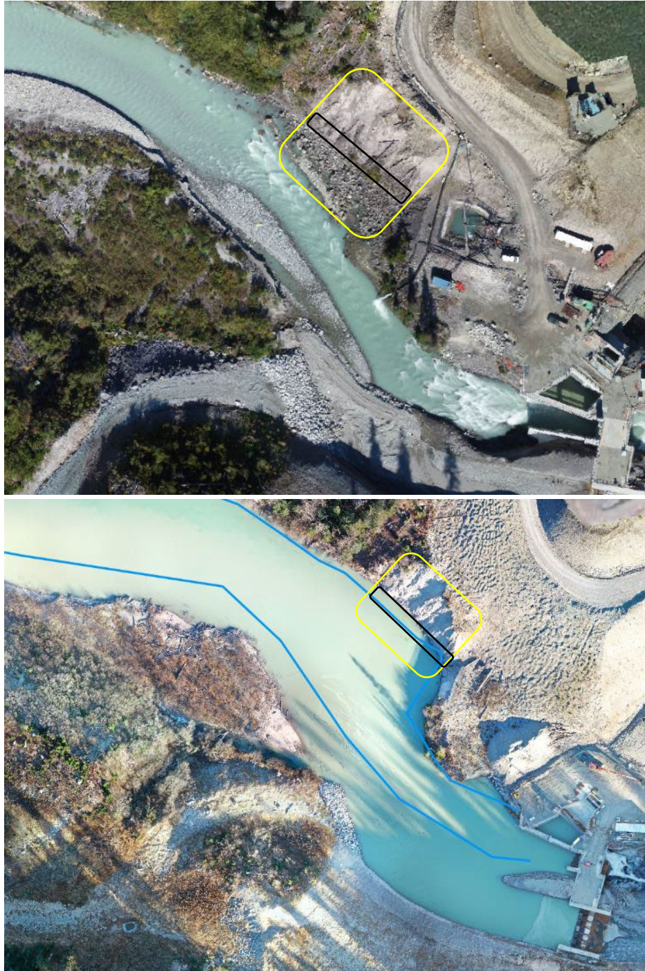
Figure 4. Upper Lillooet River Upstream Reach displaying river left bank erosion in headpond (yellow outline) in 2023 (bottom) in comparison to 2016 (top). Toe of slope outline in black has moved upslope due to water level rise and is no longer protected from flow erosion by larger cobble boulders bar causing some erosion on steep left bank into the headpond. Blue outline displays 2016 channel path for visual representation.
