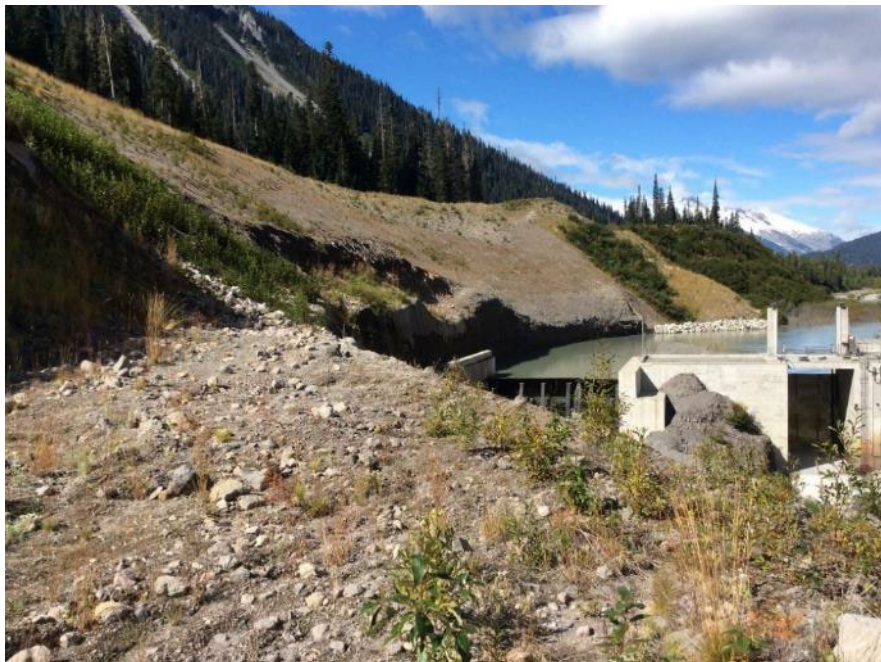
Figure 16. Looking upstream at the dam from ULL-PRM02 on September 01, 2020.
