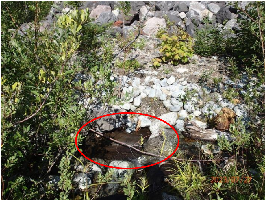
Figure 38. Exposed geotextile within the stream channel at ULL-ASTR04 on July 27, 2023.
