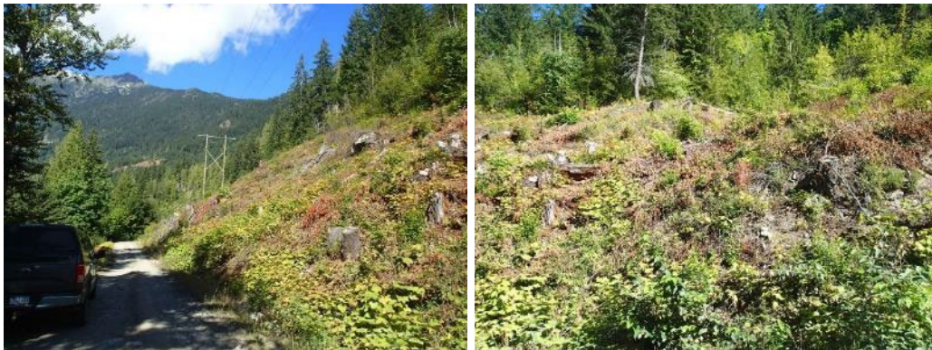
Figure 35. Vegetated screen along the transmission line at ULH-MAMCM21, assessed on August 25, 2020.
