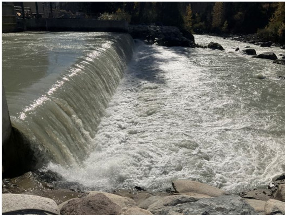
Figure 12. Looking RR-RL at ULL-TAILWQ on October 06, 2023.
