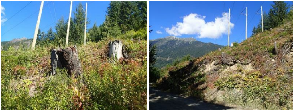
Figure 38. Vegetated screen along the transmission line at ULH-MAMCM22, assessed on August 25, 2020.
