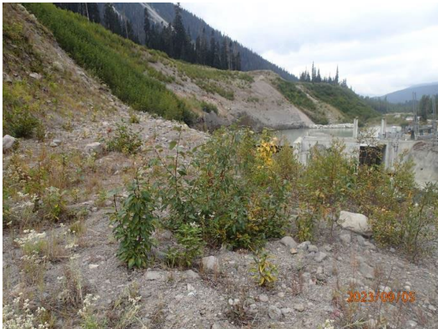
Figure 18. Looking upstream at the dam from ULL-PRM02 on September 05, 2023.
