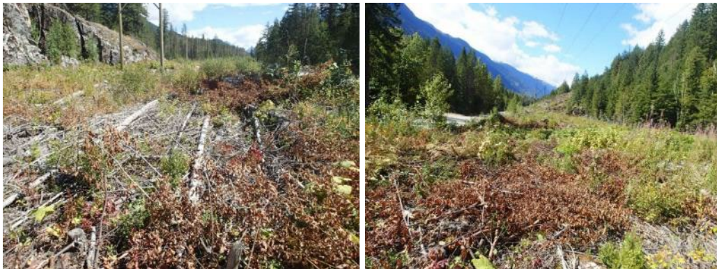
Figure 23. Vegetated screen along the transmission line at ULH-MAMCM12, assessed on August 24, 2020.
