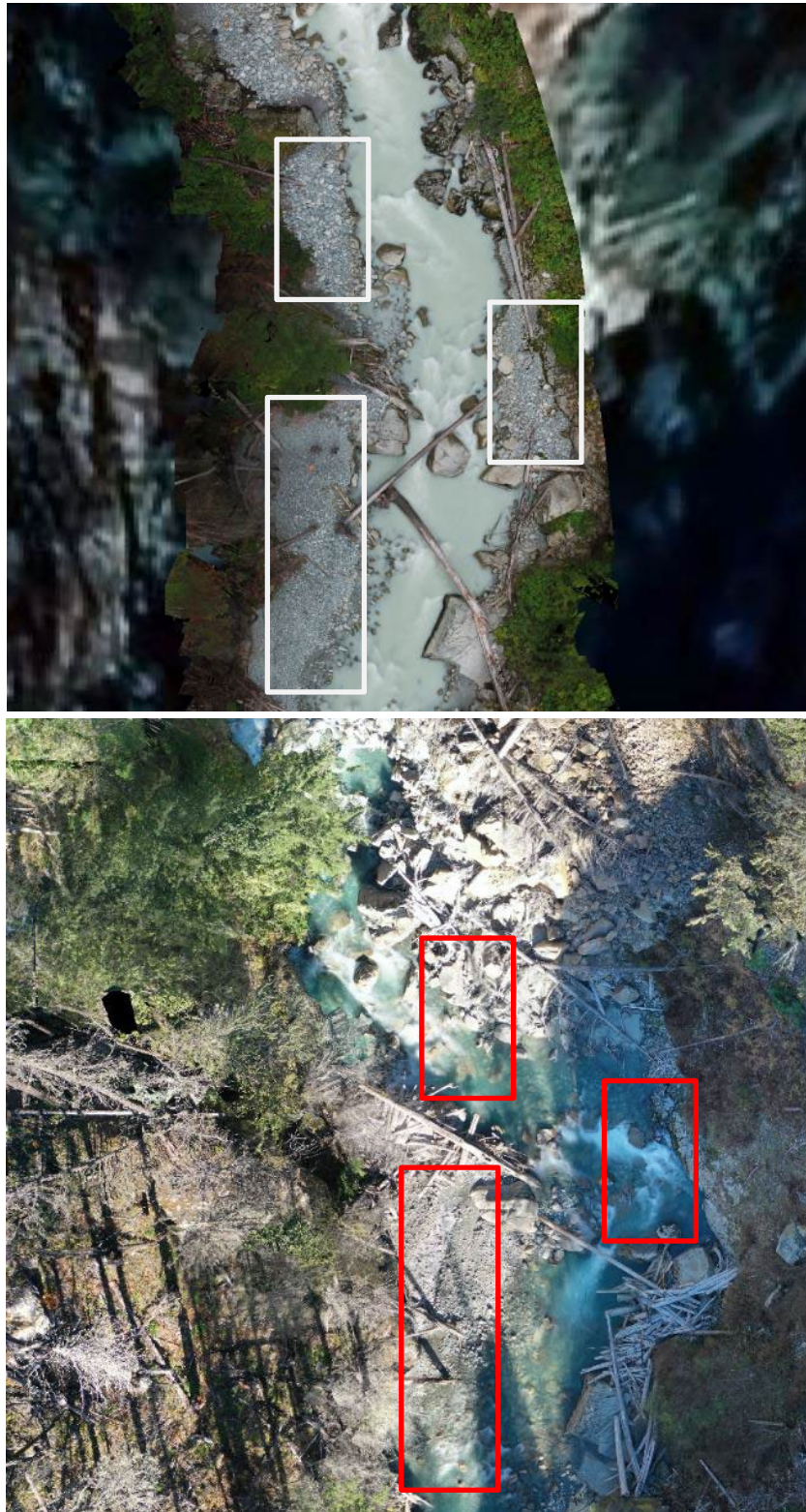
Figure 3. Boulder Creek Upstream Reach displaying shift in channel path caused by landslide. Channel in 2023 (bottom) has higher sinuosity than in 2016 (top) causing scour of gravel outlined in red along the margins of the channel.
