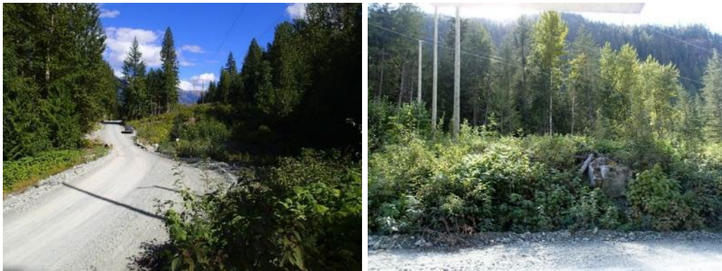
Figure 29. Vegetated screen along the transmission line at ULH-MAMCM17, assessed on August 24, 2020.
