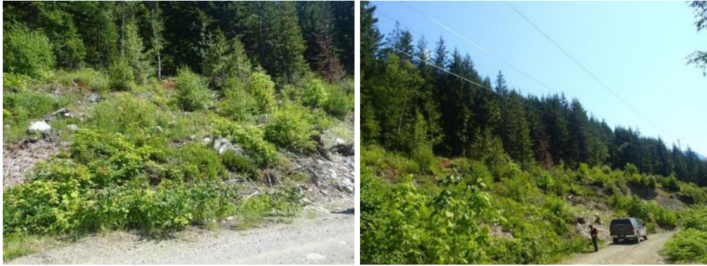
Figure 43. Vegetated screen along the transmission line at ULH-MAMCM24, assessed on June 19, 2018.
