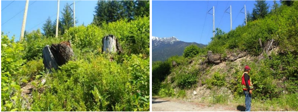
Figure 37. Vegetated screen along the transmission line at ULH-MAMCM22, assessed on June 19, 2018.
