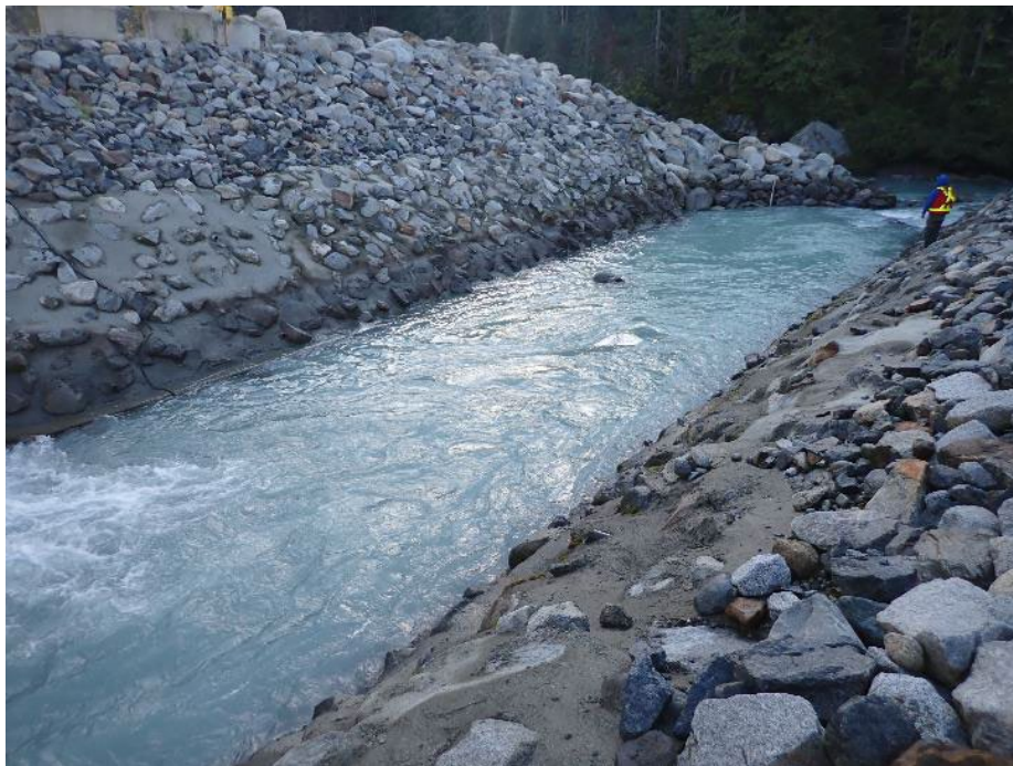
Figure 4. Looking downstream from river right at BDR-TRAG01 on October 03, 2023.
