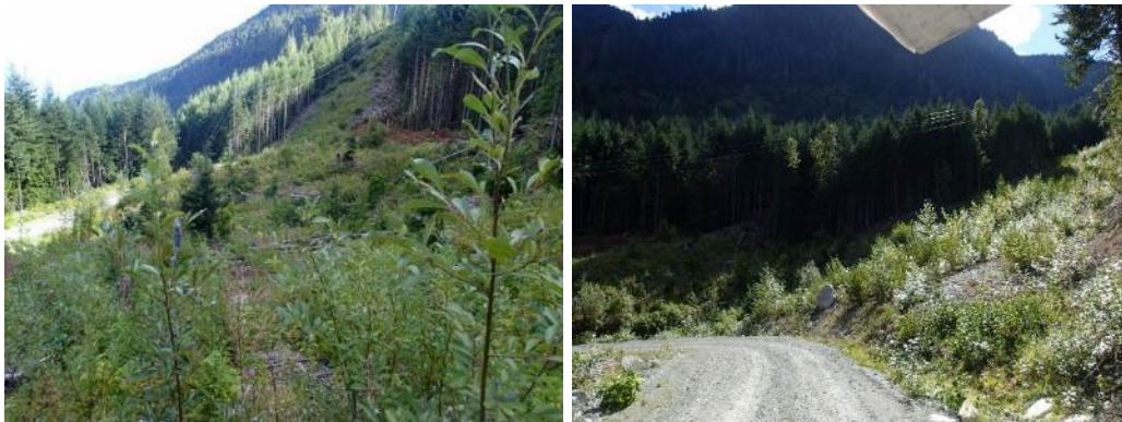
Figure 50. Vegetated screen along the transmission line at ULH-MAMCM27, assessed on August 25, 2020.
