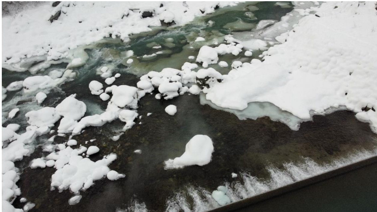
Figure 14. View of Upper Lillooet diversion reach at the tailrace confluence on December 22, 2022.
