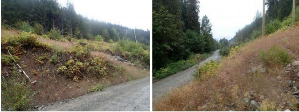
Figure 16. Vegetated screen along the transmission line at ULH-MAMCM09, assessed on June 14, 2018.
