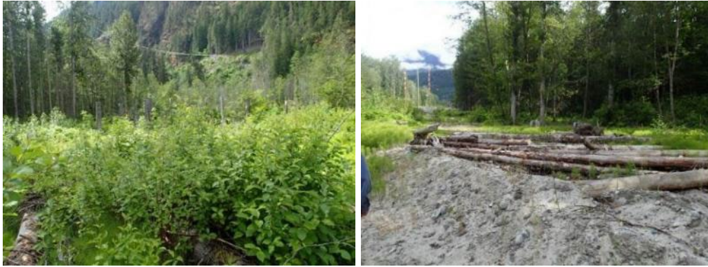
Figure 25. Vegetated screen along the transmission line at ULH-MAMCM14, assessed on June 6, 2018.
