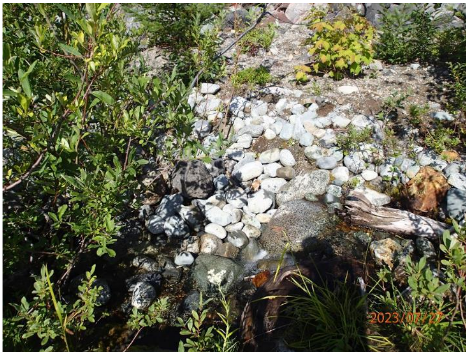
Figure 39. Location where geotextile had been exposed adjacent to the stream channel, after covering exposed section with cobble by hand, on July 27, 2023.
