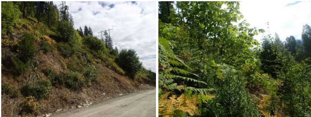
Figure 14. Vegetated screen along the transmission line at ULH-MAMCM08, assessed on August 24, 2020.
