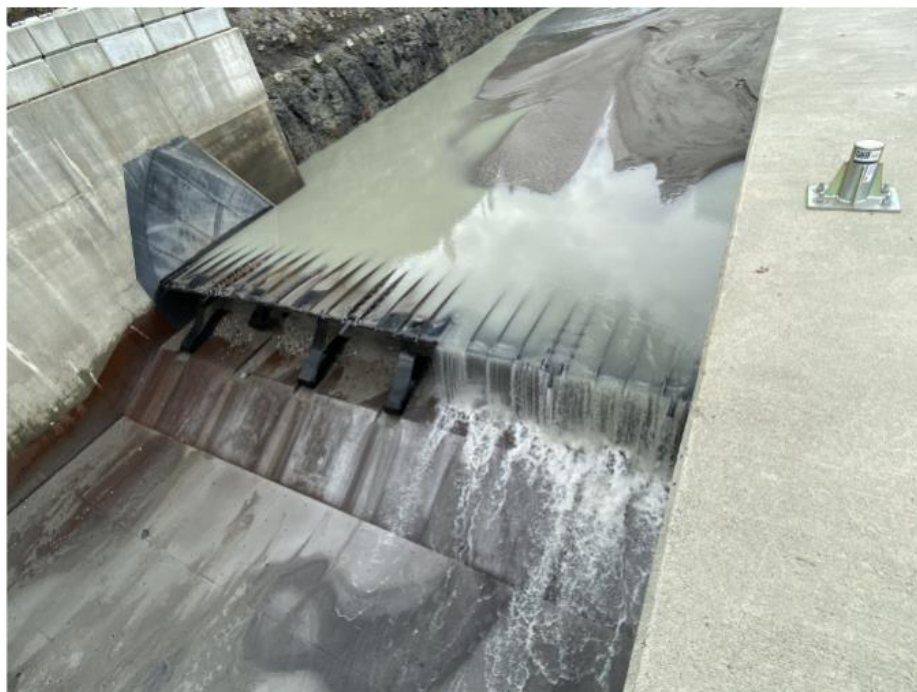
Figure 18. Obermeyer weir fully lowered during peak flow event to convey accumulated headpond sediment to be flushed downstream on June 29, 2023.
