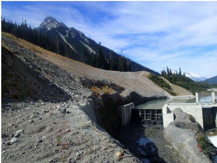
Figure 14. Looking upstream at the dam from ULL-PRM02 on September 07, 2018.
