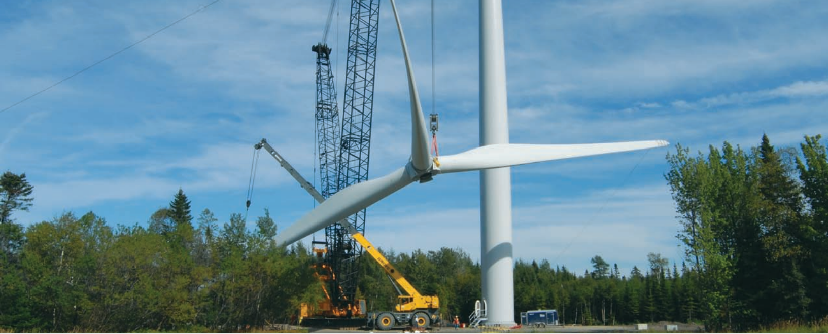
Wind turbine installation
