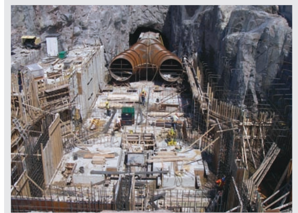
Construction at Umbata Falls hydroelectric facility
