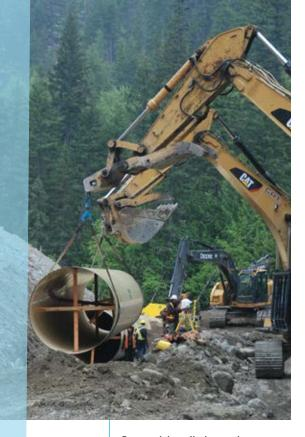
Penstock installation at the Kwoiek Creek hydroelectric project in British Columbia.
